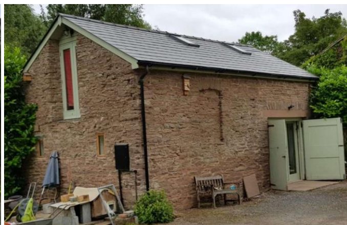
The building in 2021 without flue
